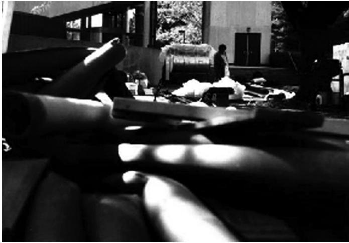
Fig. 5. The dismantling of the informal settlement.
